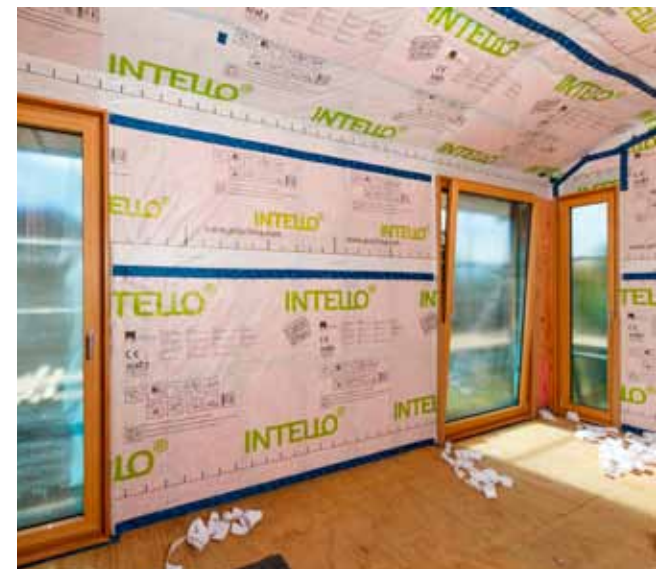
Fig. 1: Intello used between insulation and plasterboard.
