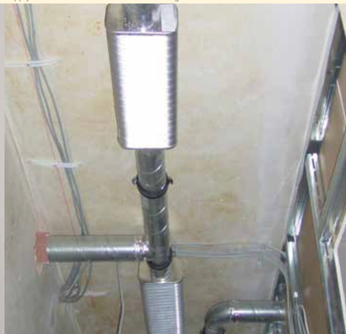
Supply air ducts with sound absorbers during installation
