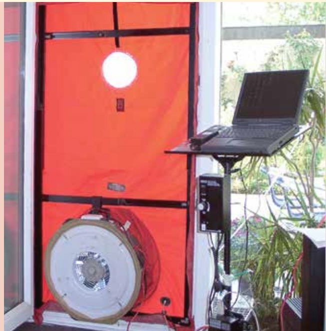
Fan for an air pressure test
