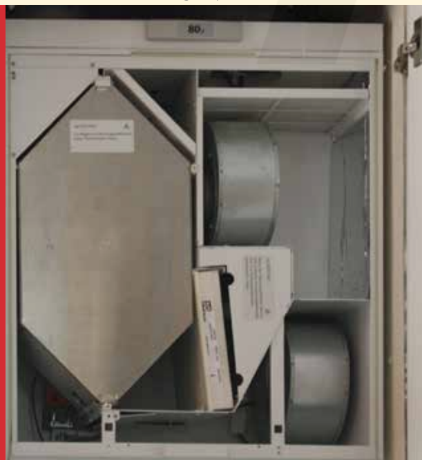
Ventilation unit with heat exchanger exposed
