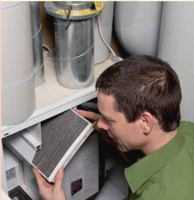
Replacing the filter of a ventilation unit.
