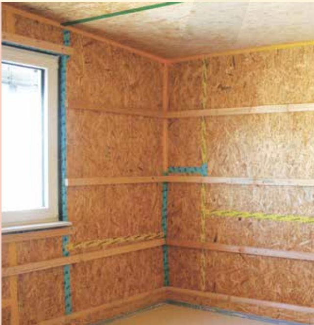
Airtight connections between wood composite boards
